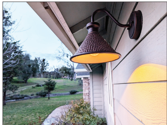
An example of a fully shielded light fixture.
