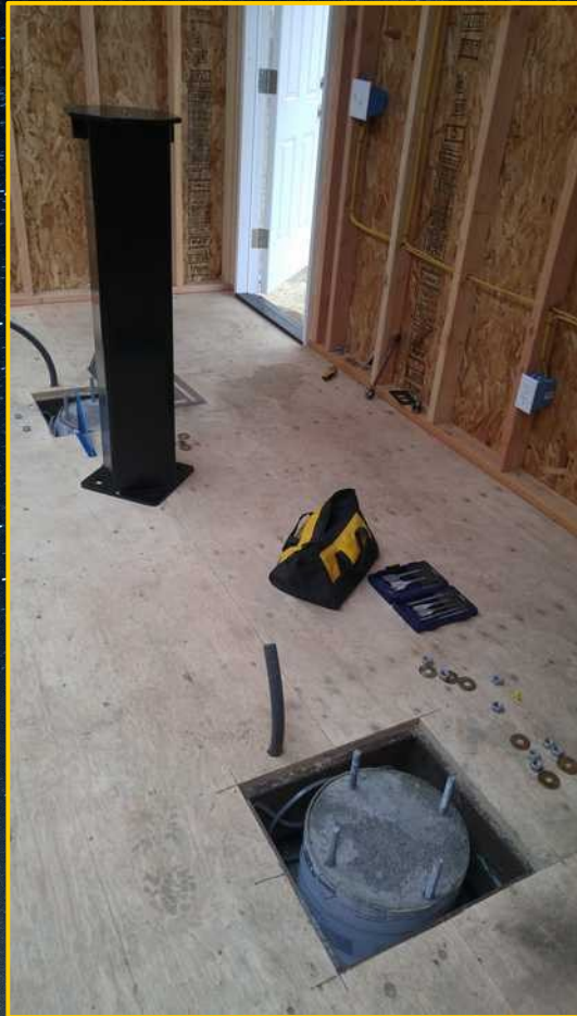
North Pier Installation
