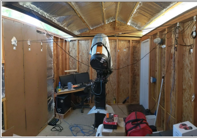
Figure 2. Observatory Sensor Wiring. Note Masonite Panels and Reflectix on Left (West) Wall.
