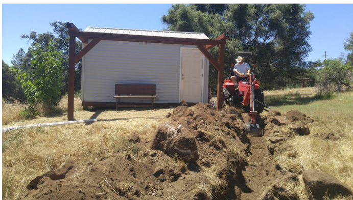
Ethernet Trenching Nearly Done - Those Rocks Were Terrible!
