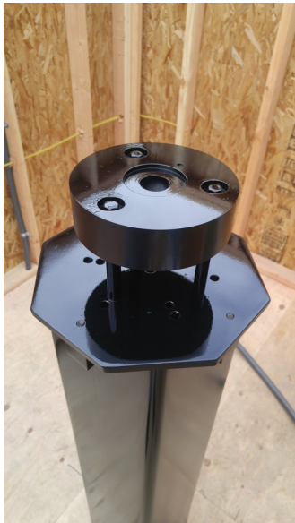
North Pier Installed, With Custom CGEM Adapter
