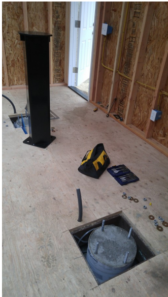
Pier Footings and Pier (North at Top)
