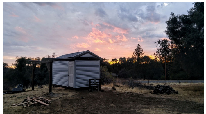
Nightfall, Build Day 3. The Observatory is Nearly Complete!
